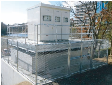
* The lower structure was raised to allow for easy observation of the bearings.
