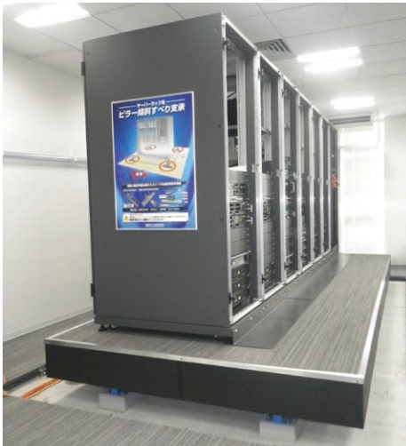
* The flooring surrounding the server location was removed to allow for easy observation of the bearings.
